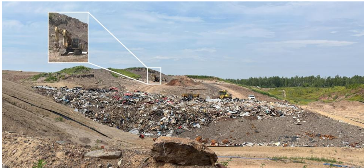
Figure 2-7: General Waste Magnet Attachment
