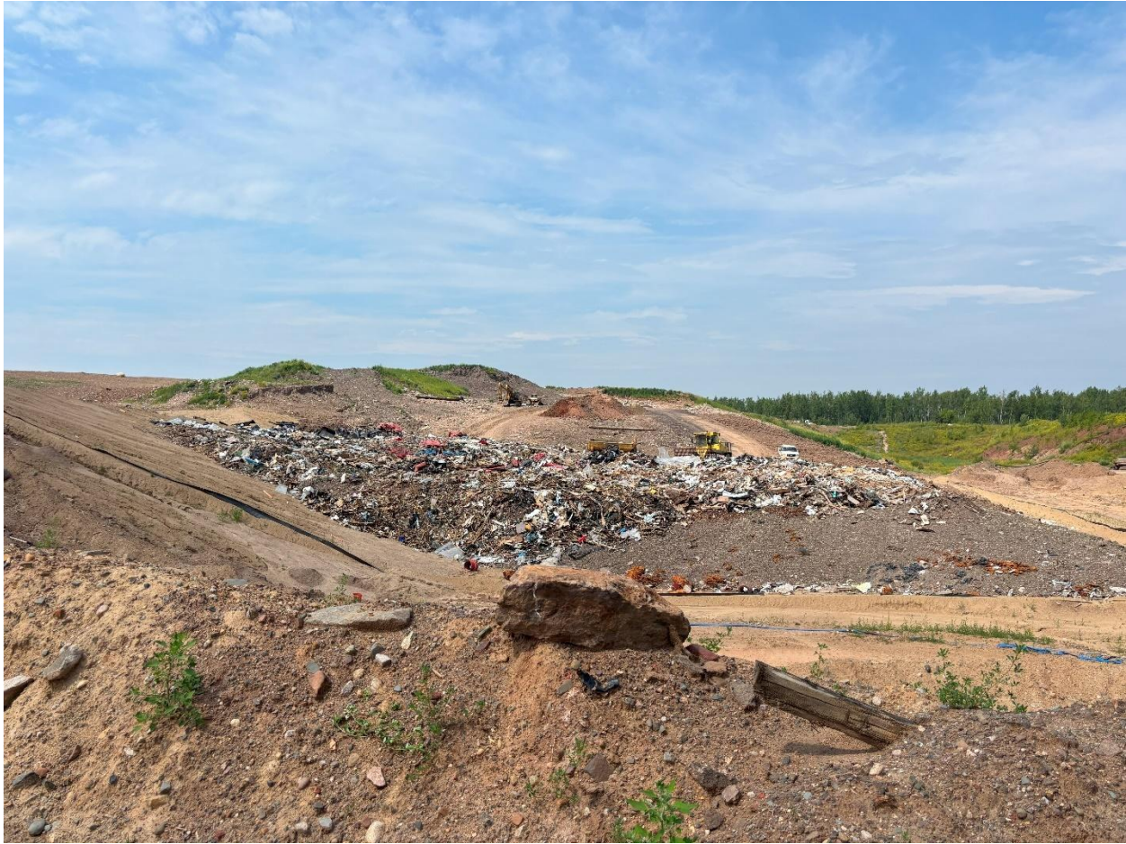
Figure 2-2: General Waste Landfill, SW-620
