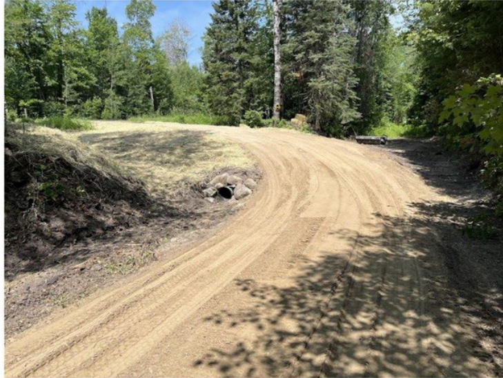
Phase 1 construction on the Wilderness ATV Trail.
