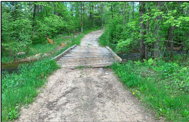
Old Balsam Creek Bridge before replacement.
