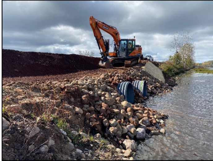
Construction and culvert replacement on the Alborn Trail.
