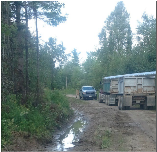
Logging road maintenance project.
