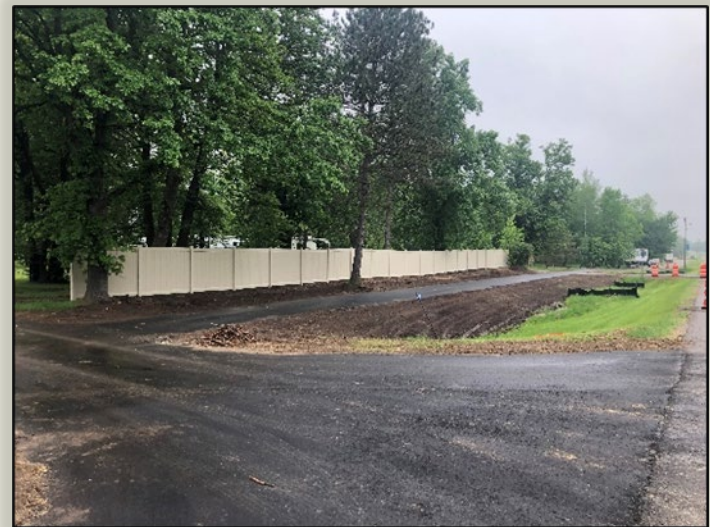
Construction of Squaw Lake Connector Trail.
