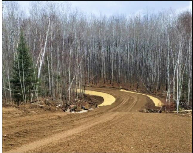
Len Hardy Memorial Trail Construction.
