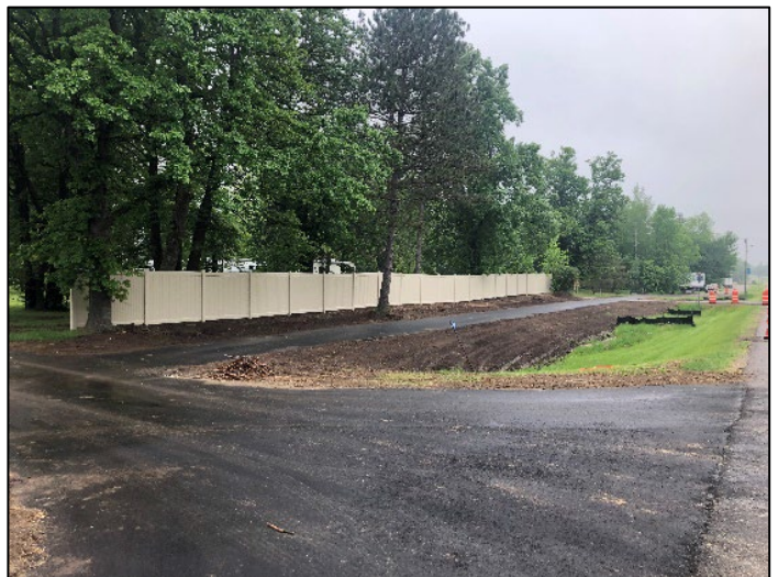
Squaw Lake Connector Trail Construction.
