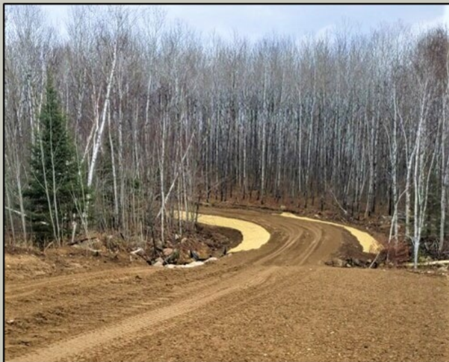
Construction activities on Len Hardy Trail.
