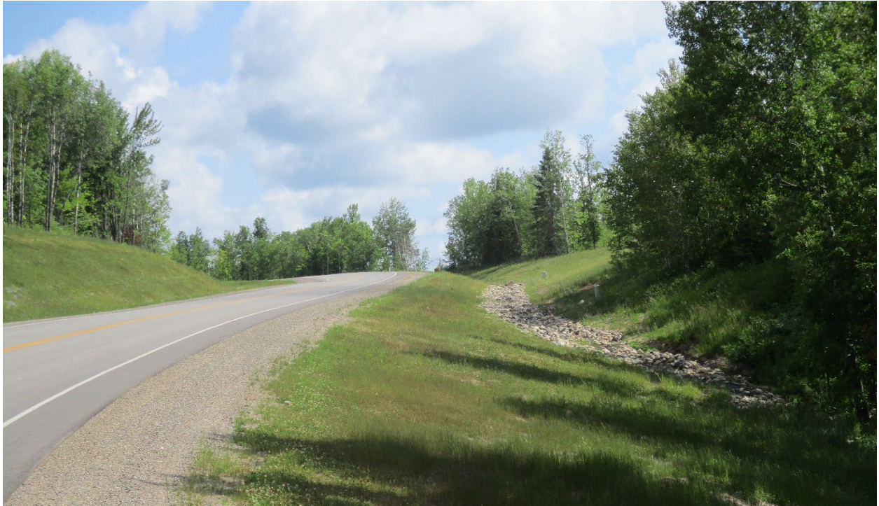
CSAH 7 Reconstruction from Hwy 169 to 1.3 miles north
