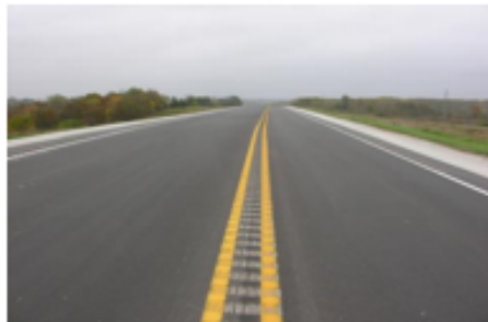
Centerline Rumble Strips
