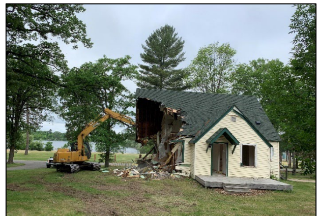
Demolition of Fairground Caretaker House.
