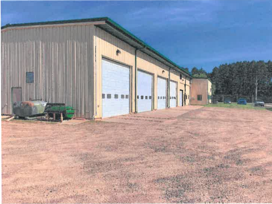
Southeast Side of Land Building – Garage Bays
