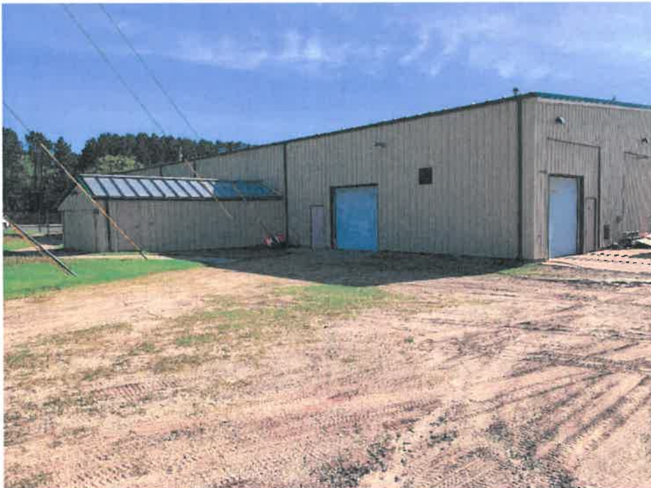
Southwest Side of Land Building – Garage and Storage Bays
