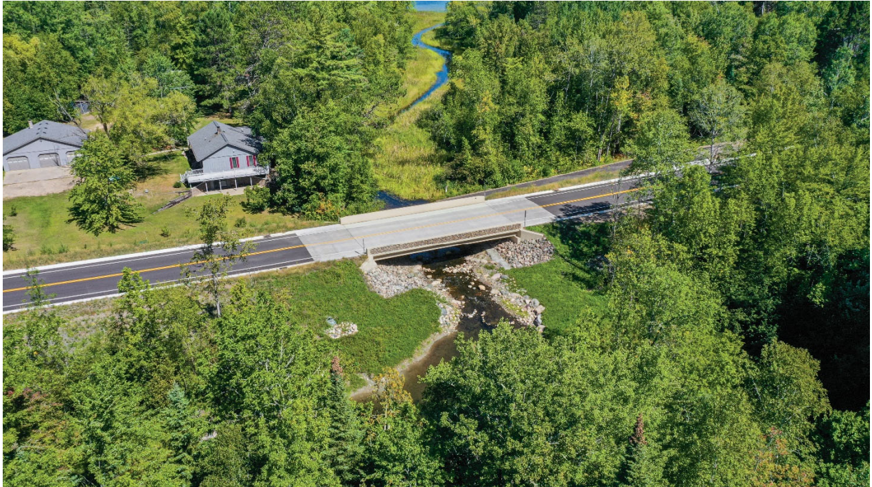
Bridge replacement on CSAH 60 which was part of the road reconstruction project from CSAH 49 to Willow Creek Trail
