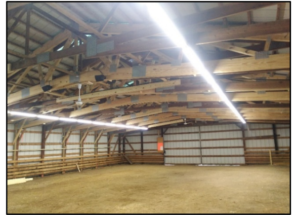
Repaired cattle barn at Fairgrounds.
